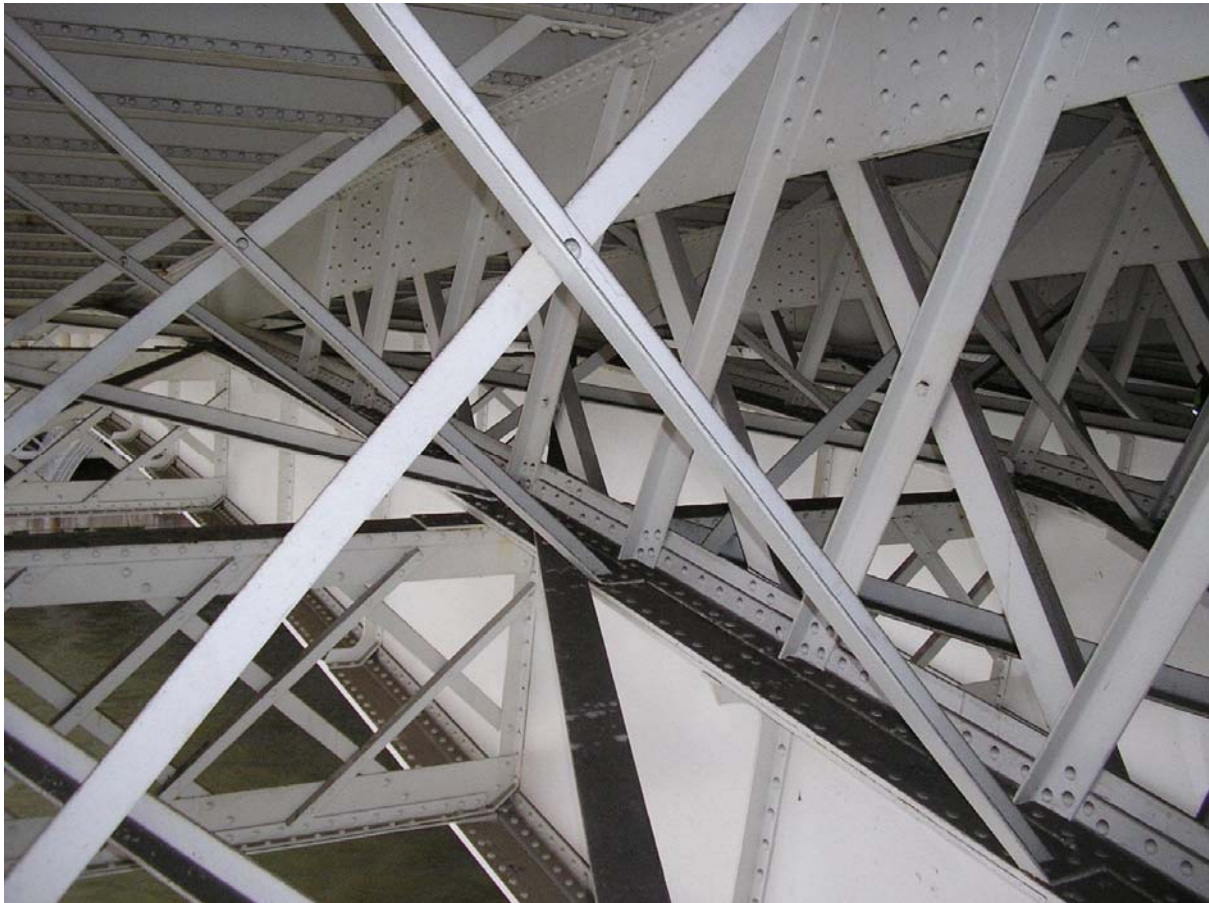
Figure 3. Braces between arch ribs
