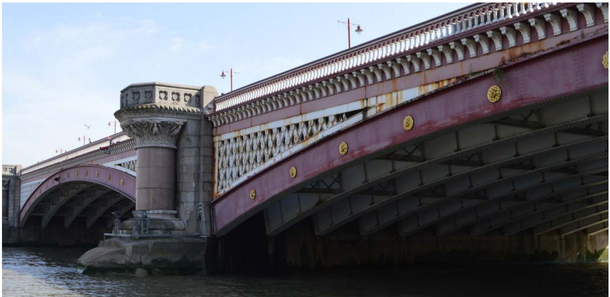
Figure 157. Current rust staining on the bridge
