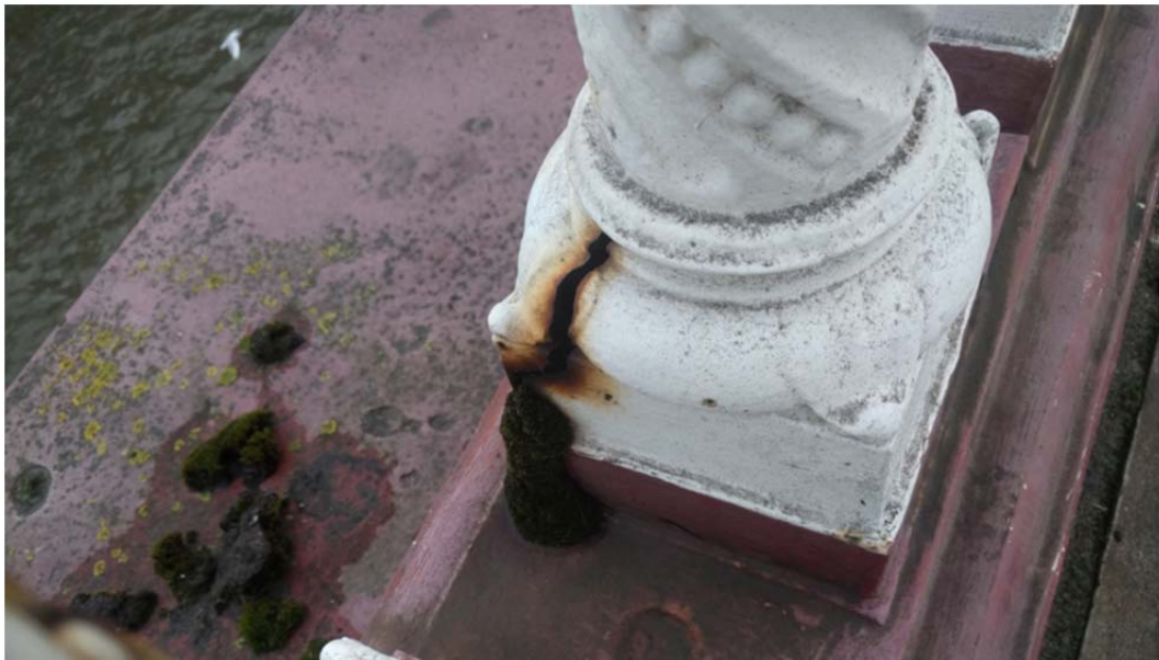
Figure 4. Example of large crack in the corner of baluster base that is required to be filled with epoxy filler.
